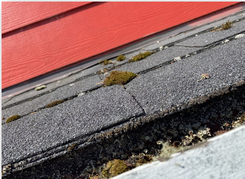
Upper floor exterior egress stair. Roofing is nearly at end of design life and should be replaced. Siding repairs, paint, and recaulking needed soon.
