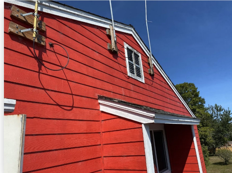
Upper floor exterior egress stair. Roofing is nearly at end of design life and should be replaced. Siding repairs, paint, and recaulking needed soon.
