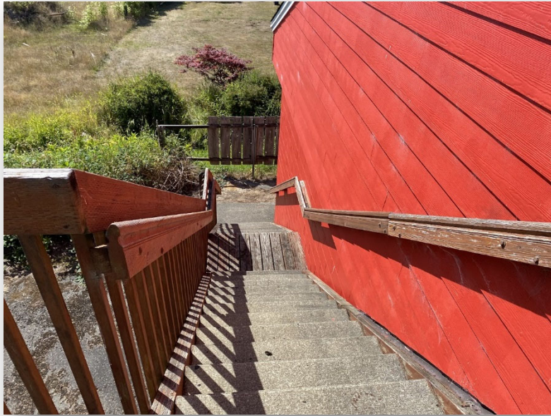
Upper floor exterior egress stair. Roofing is nearly at end of design life and should be replaced. Siding repairs, paint, and recaulking needed soon.
